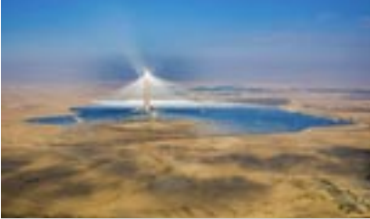
Ashalim solar power station in the Negev desert. (Yonatan Sindel/Flash90)
