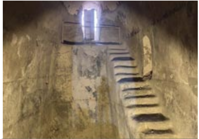
Large Water Cistern
