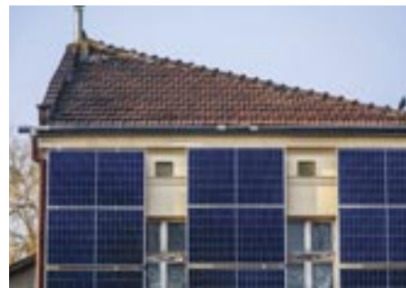
A number of solar collector panels are attached to the front wall of an old house in the center of Krakow, Poland. (Beata Zawrzel/NurPhoto via Getty Images)
