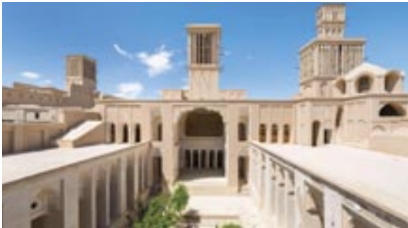
The openings of the towers face the prevailing wind, catching it and funneling it down to the interior below (Credit: Alamy)
