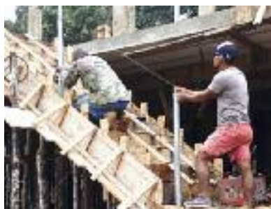
Constructing the staircase
